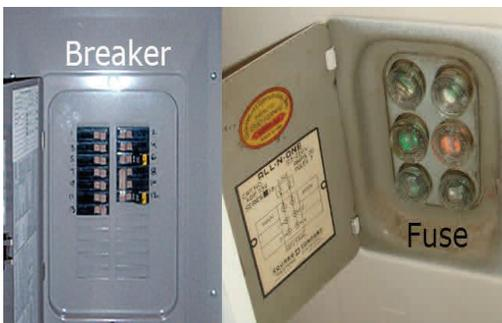
not the least of which is how quickly they can be reset. It is usually clear which switch has tripped, and it can be easily reset in most cases. For the average homeowner, it is also safer because there is no question about choosing the right fuse rating and all of the electrical connections are hidden in a breaker box.
