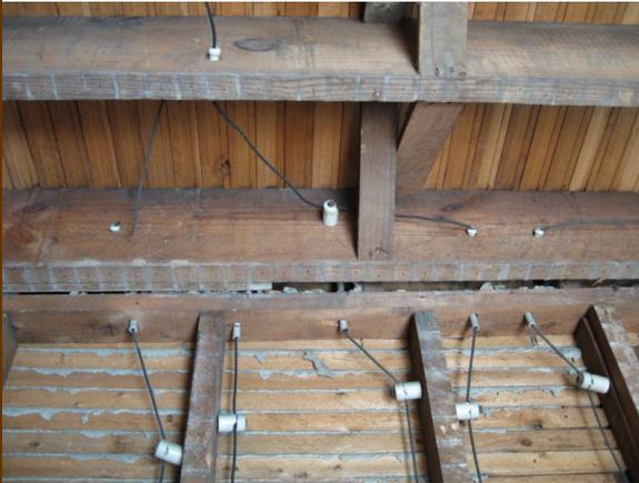
the single-conductor wires were supported by cylindrical ceramic nailed-down knobs, and passed through studs or joists via ceramic insulating tubes. Splices were sometimes made by soldering wires together and then wrapped up with cloth tape, and just left in “open air” without the splice being contained in an electrical box. Where conductors would come into a switch box, the wires would be protected with cotton cloth saturated with asphalt, called “loom”.
